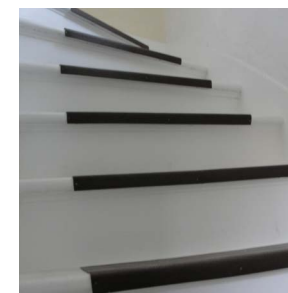
After lead paint interim controls
